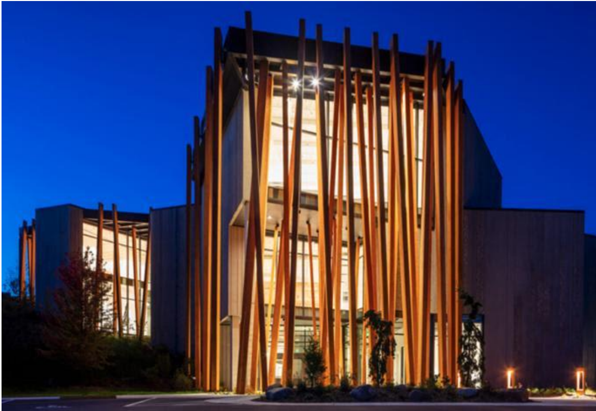
Exterior of The John Michael Kohler Art Preserve in Sheboygan. Courtesy of John Michael Kohler Arts Center, Sheboygan, Wisconsin. Photo: Durston Saylor.
